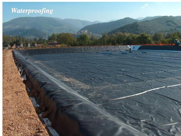
**Figure 20** Impermeable soil cover.
